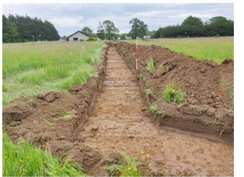
Plate 16: Phase II Testing; Trench 3 from W
